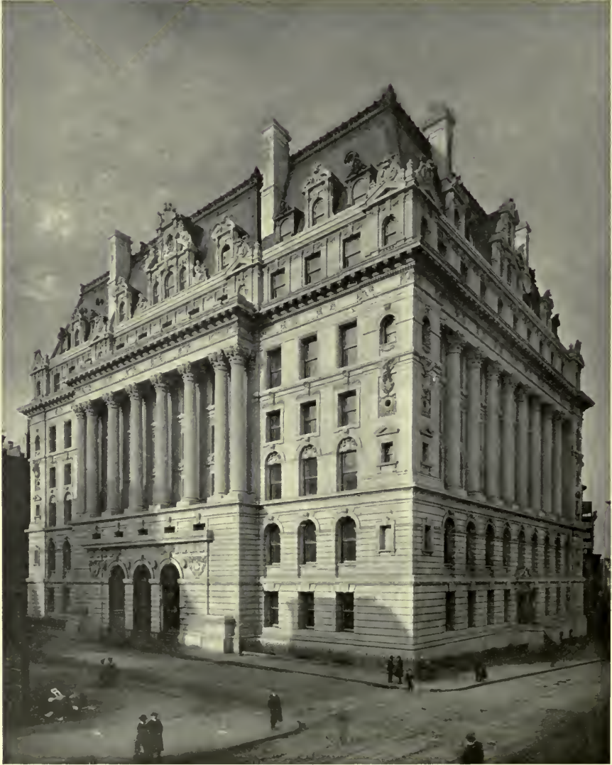
THE NEW "HALL OF RECORDS." Chambers and Centre Streets, New York City. The late J. R. Thomas, Architect.
